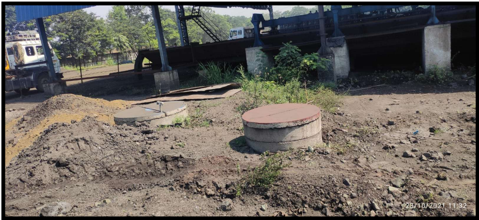
Pit No. 4 (Near Rolling Mill)
