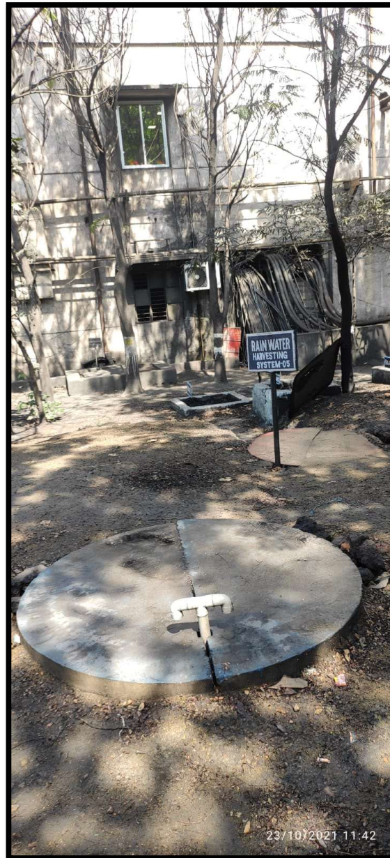
Pit No. 5 (Near Power Plant)
