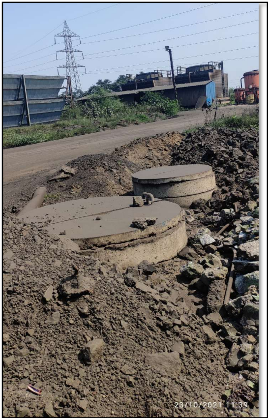
Pit No. 3 (Near ferro alloys unit)
